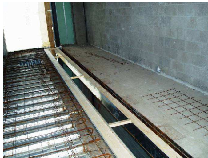
Figure 13 - Expansion Joint Section Photo Courtesy Jim Boje, PE (Wendel)
